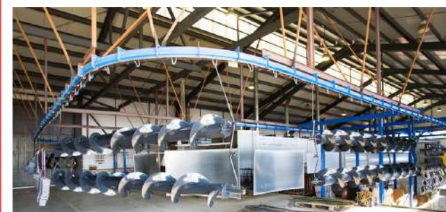
Powder Coating Facilities
